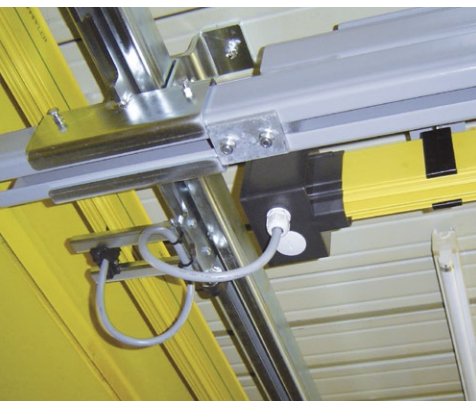
Combined reliability with enclosed conductor rail to an equipment bridge .
