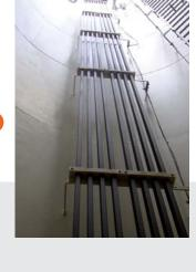
Towerbuss for Down-Tower Power Transmission
